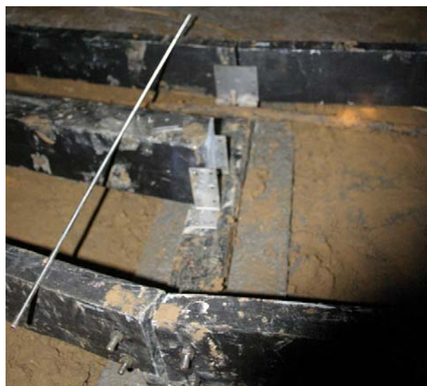
Painted, sealed stringers being assembled. Four bolts can be used to attach handrail post if required. Note detail on replacement stringer
