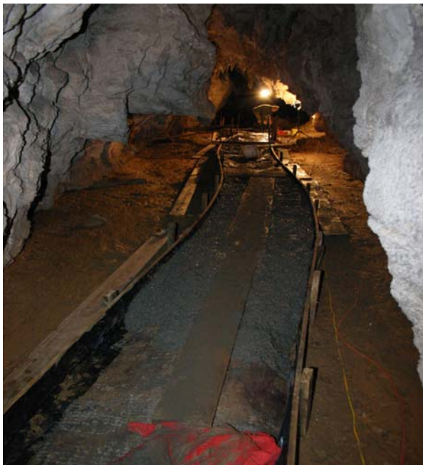
Laying Concrete in the cave
